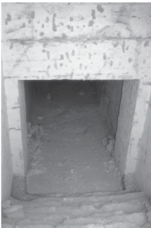
Figure 2: Steps leading into WV 25. Note unusual lip at the bottom of the stairs.
